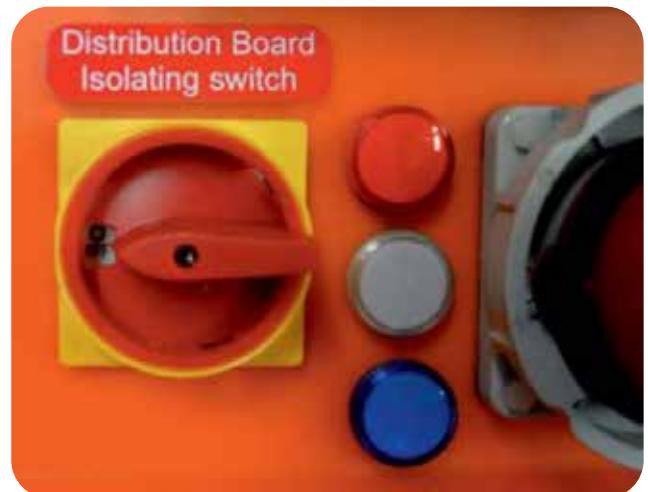
Powersafe clearly mark the main switch. As an added feature Powersafe fit coloured indicator lights to show power on each phase.
