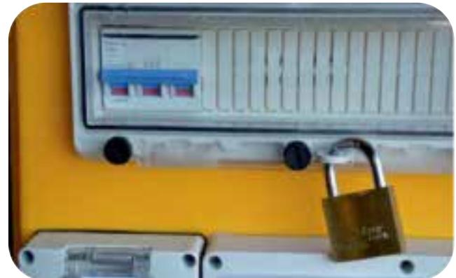
By locating a main isolator behind a pad-lockable window, as some of our competitors do, where it can be secured in an open position, meets clause (b) of the standard, but fails to meet clause (c).
